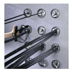
TDUX is a unique inflatable wraparound duct sealing system for permanently sealing telephone cable ducts in order to prevent the leakage of water from the duct into exchange vaults or manholes. It has been developed for use with plastic, concrete or steel ducting wall-feedthrough systems. It can be used with polyethylene or lead-jacketed cables.
